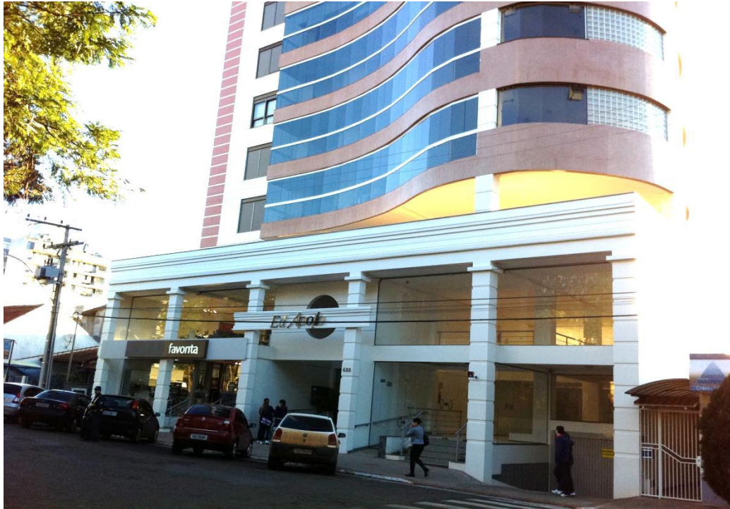
Figura 25: Vista parcial – Fachada Principal
